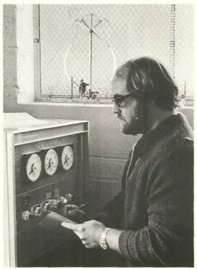
RALPH RUSK (5715) monitors a test underway with the 4.5-metre wind turbine at a test site near Bldg. 899, about a mile east of Tech Area 1. Data will contribute to the design of a new 17-metre wind turbine.
